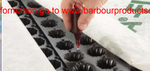
Joining sheets with DELTA®-FLORAXX connecting elements.
